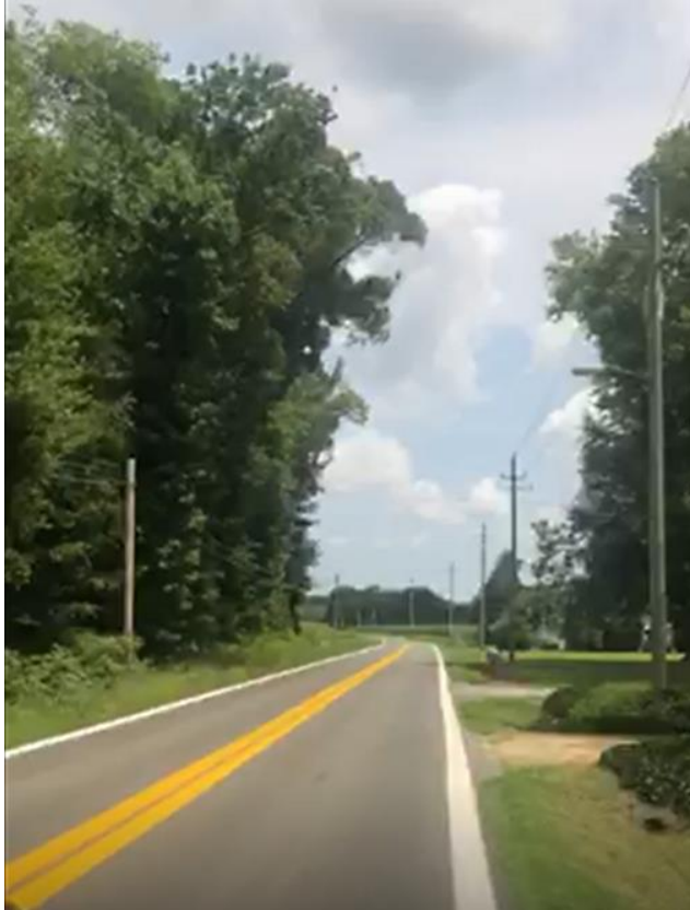
White and yellow striping widened from 5' to 10"
