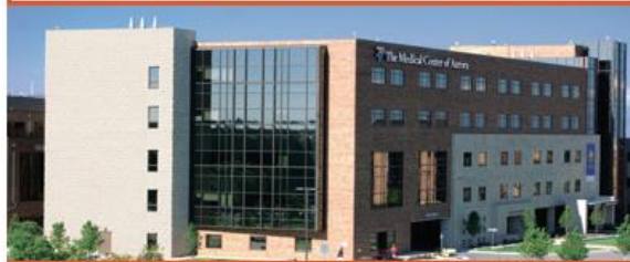
The Medical Center of Aurora Spalding Rehabilitation Center
