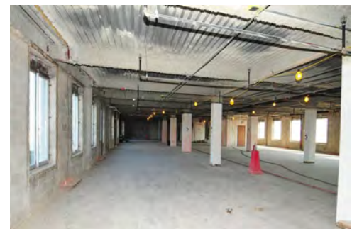
Hull Building during renovation
