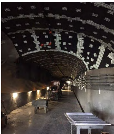
Construction of the underground tunnel
