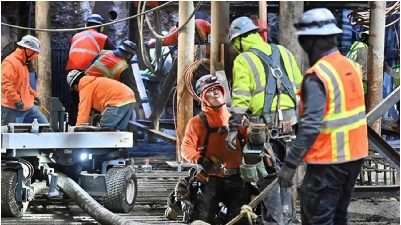
More than 2,500 people have worked to complete this project
