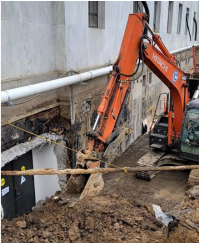
36,000 cubic yards of materials were excavated from the ground (G) level
