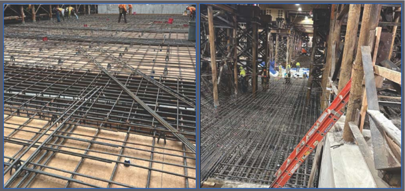
5,406,000 lbs. of rebar has been installed.
