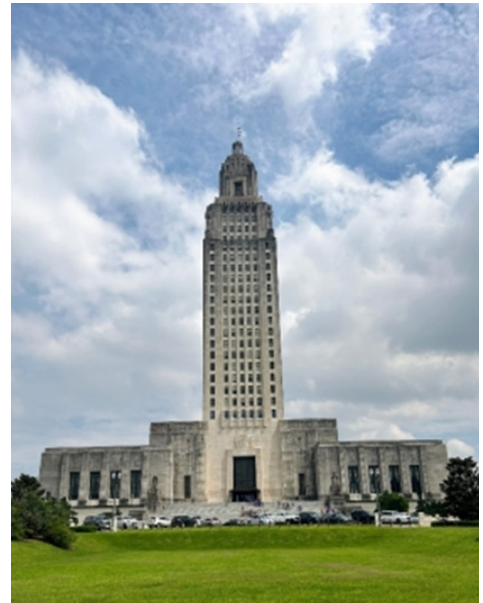
The Capitol building
