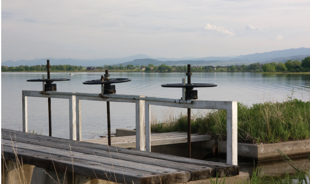
Headgates and outlet to Lonetree Reservoir in Colorado.
