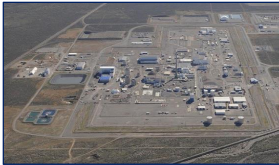
Idaho Nuclear Technology and Engineering Center
