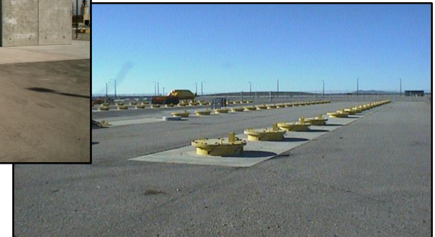
Underground vault storage
