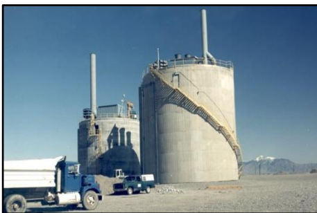
Calcine Bin Sets
