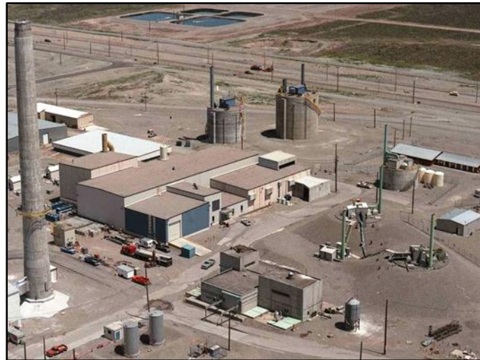
Calcine Solids Storage Facility
