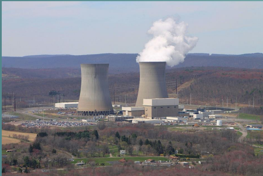
Susquehanna Steam Electric Station 2 x 1350 MW e (2700 MW e total) Boiling Light Water Reactor
