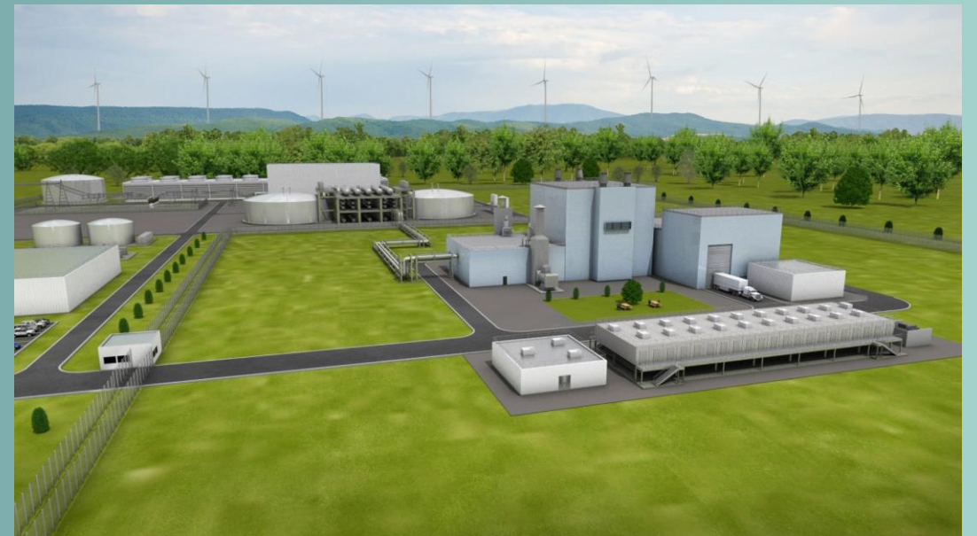
Example: TerraPower Natrium Reactor 345 MW e (with 500 MW e peak capacity) Sodium Fast Reactor with Salt Heat Storage
